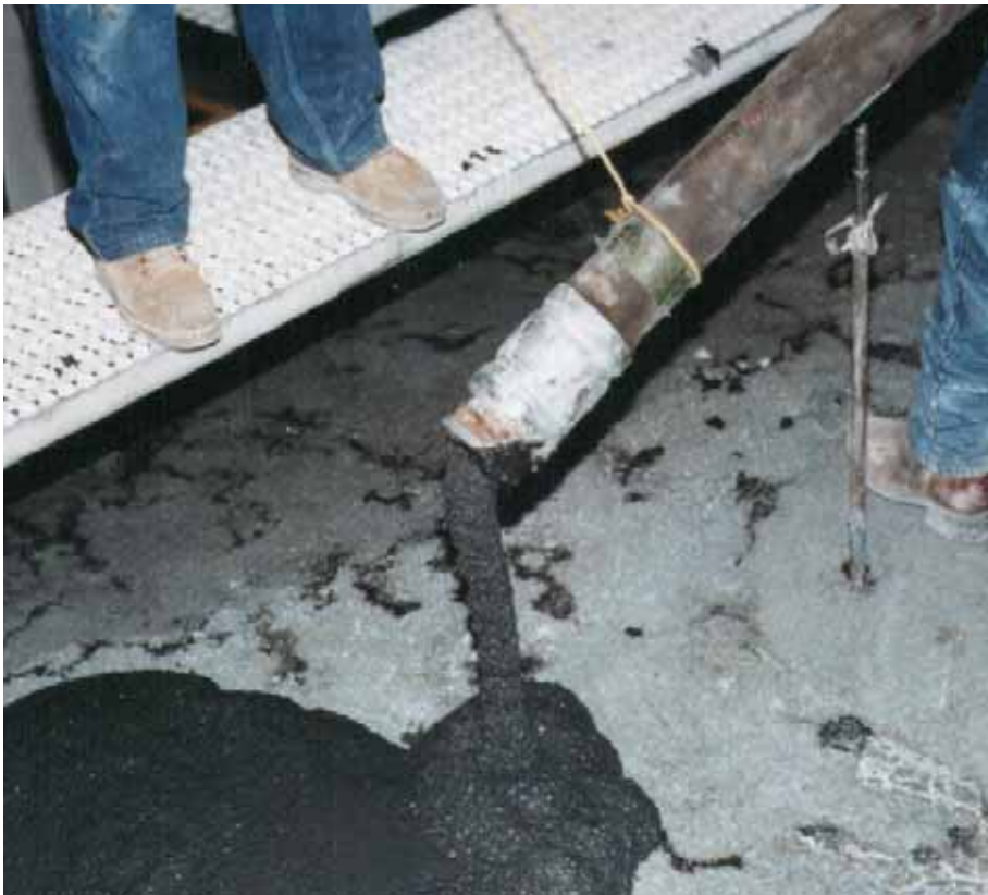
Pumping of a glass furnace crown.
