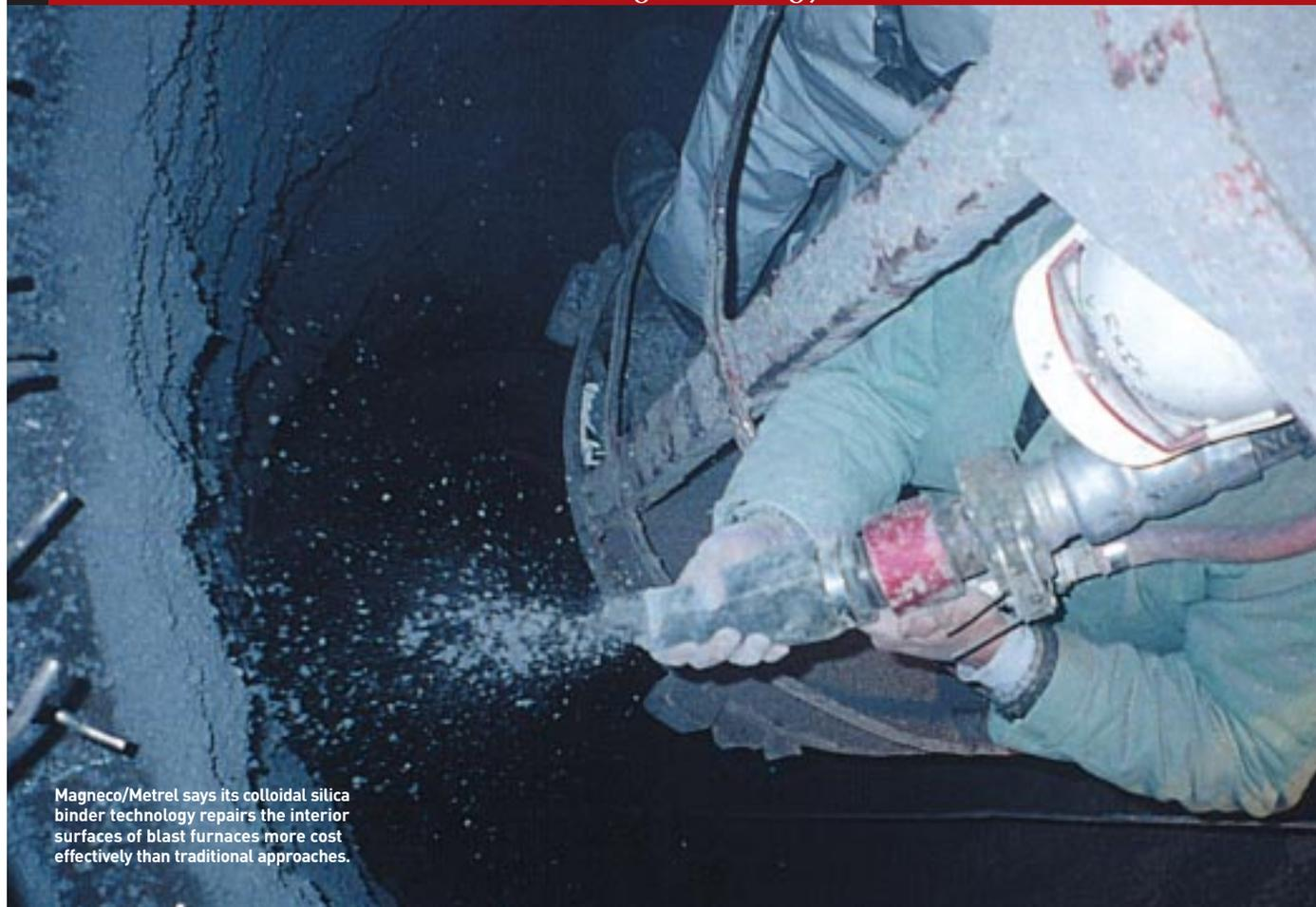
Magneco/Metrel says its colloidal silica binder technology repairs the interior surfaces of blast furnaces more cost effectively than traditional approaches.
